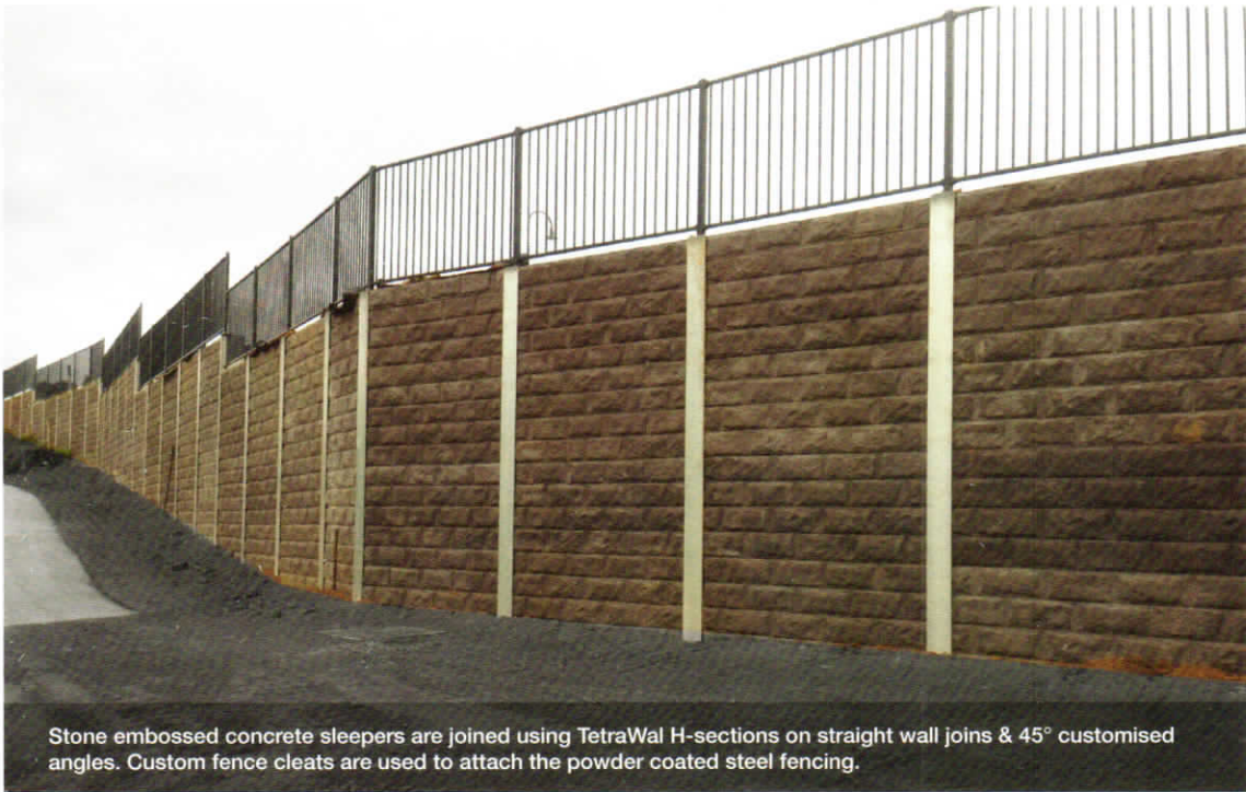
This concrete sleeper retaining wall system uses TetraWal in black Duplex (paint over galvanized steel) H-sections & 45° angles. Custom fence cleats attach the timber railing to the retaining wall.
